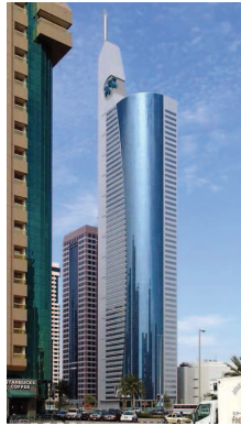
Şekil 2.2 21st Century Tower (269m.-55katlı) ,Dubai/BAE, WS Atkins and Partners [12].
