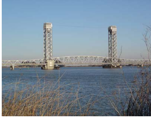
Şekil Ek 1.11 Sacramento River Bridge at Rio Vista [75].
