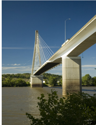
Şekil Ek 1.3 East Huntington Bridge [66].
