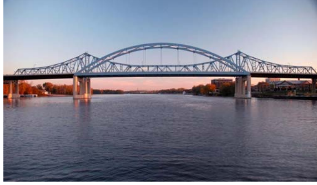
Şekil Ek 1.36 Mississippi River Bridge [102].
