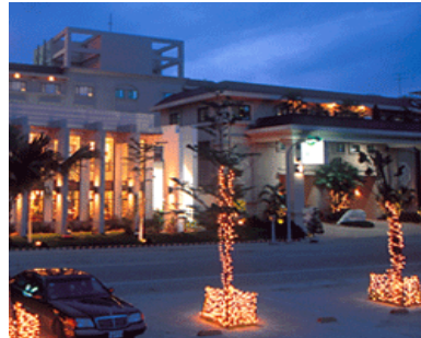
Şekil Ek 1.81 Chung Hwa Telecommunications Building [110].
