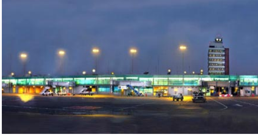
Şekil 3.30 Jorge Chavez International Airport Central Tower [25].
