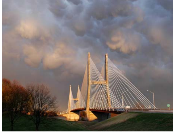
Şekil Ek 1.13 Bill Emerson Memorial Bridge [77].
