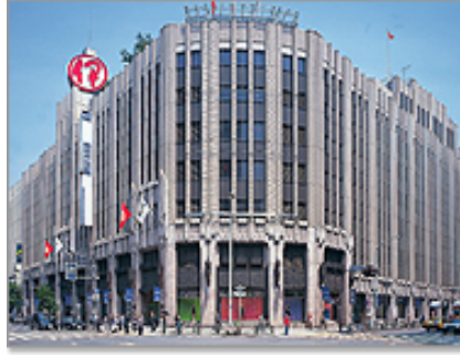
Şekil Ek 1.70 Shinjuku 3-Chome East Building [134].
