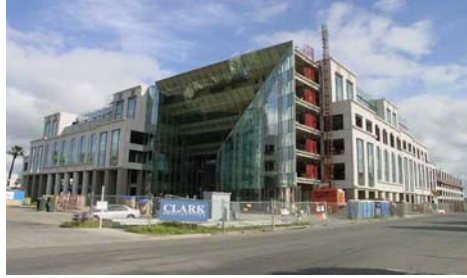
Şekil Ek 1.21 Solano County Government Building [84].
