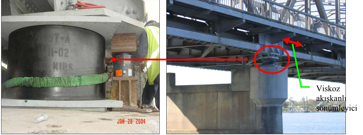
Şekil 3.11 Richmond-San Rafael Bridge [9; 10].
