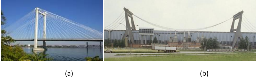
Şekil 5.32 (a) Pasco-Kennewick Bridge (b) Burgo Paper Mill, Mantova, Lombardy, İtalya (1963) [121], [369]
