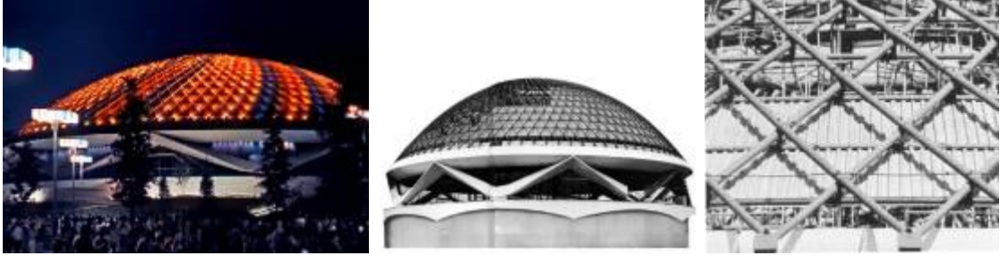
Şekil 3.154 General Electric Pavilion, New York, A.B.D (1963) [251], [252]
