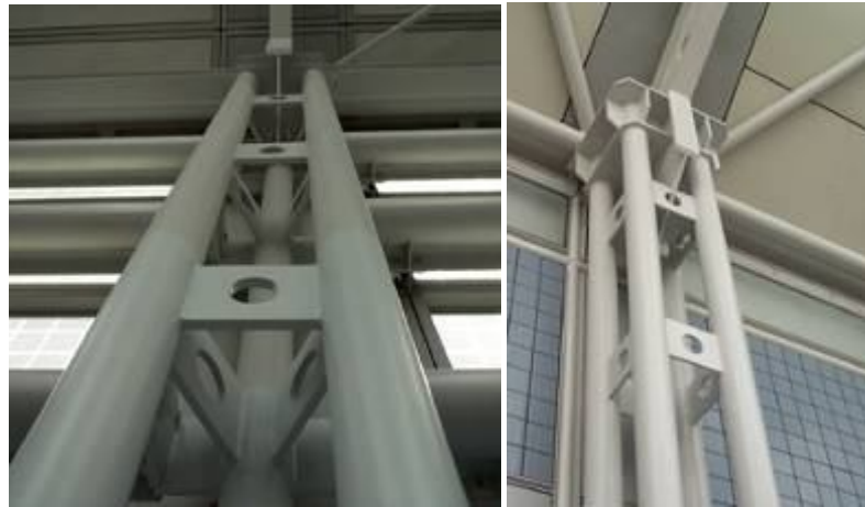
Şekil 3.41 United Airlines Terminal, Chicago, Illinois, A.B.D (1998) [96]
