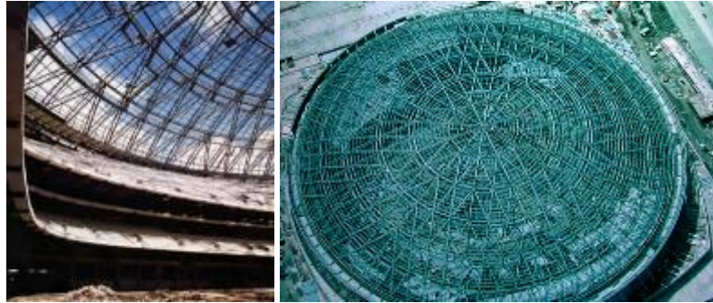
Şekil 3.151 Louisiana Superdome, New Orleans, Louisiana, A.B.D (1975) [11], [248]
