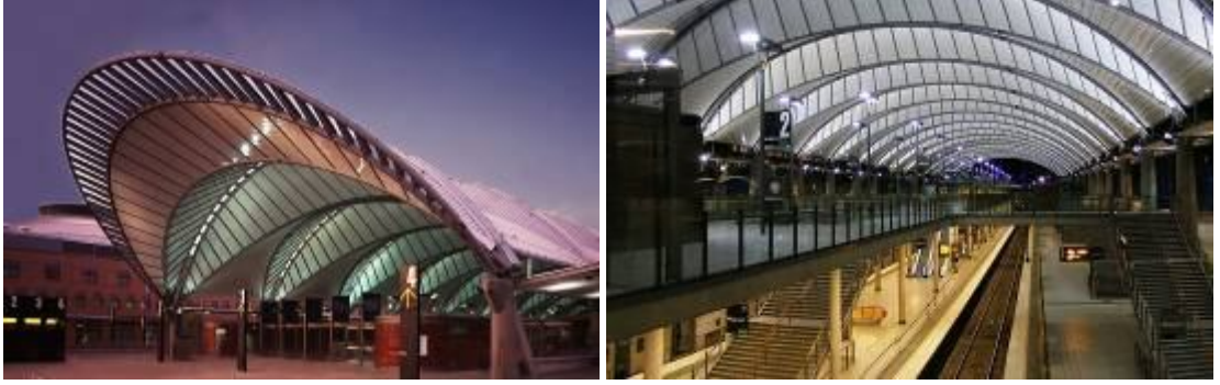
Şekil 5.5 Olympic Park Rail Station, Sydney, Avustralya (2000) [38]
