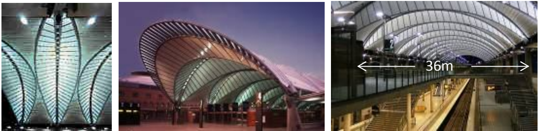
Şekil 3.9 Olympic Park Rail Station, Sydney, Avustralya (2000) [38]
