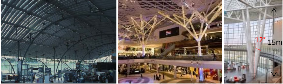
Şekil 3.34 TGV Station, France; Westfield, Londra, İngiltere(2009) ve Indianapolis Airport, Indianapolis, A.B.D (2008) [2], [88], [89]
