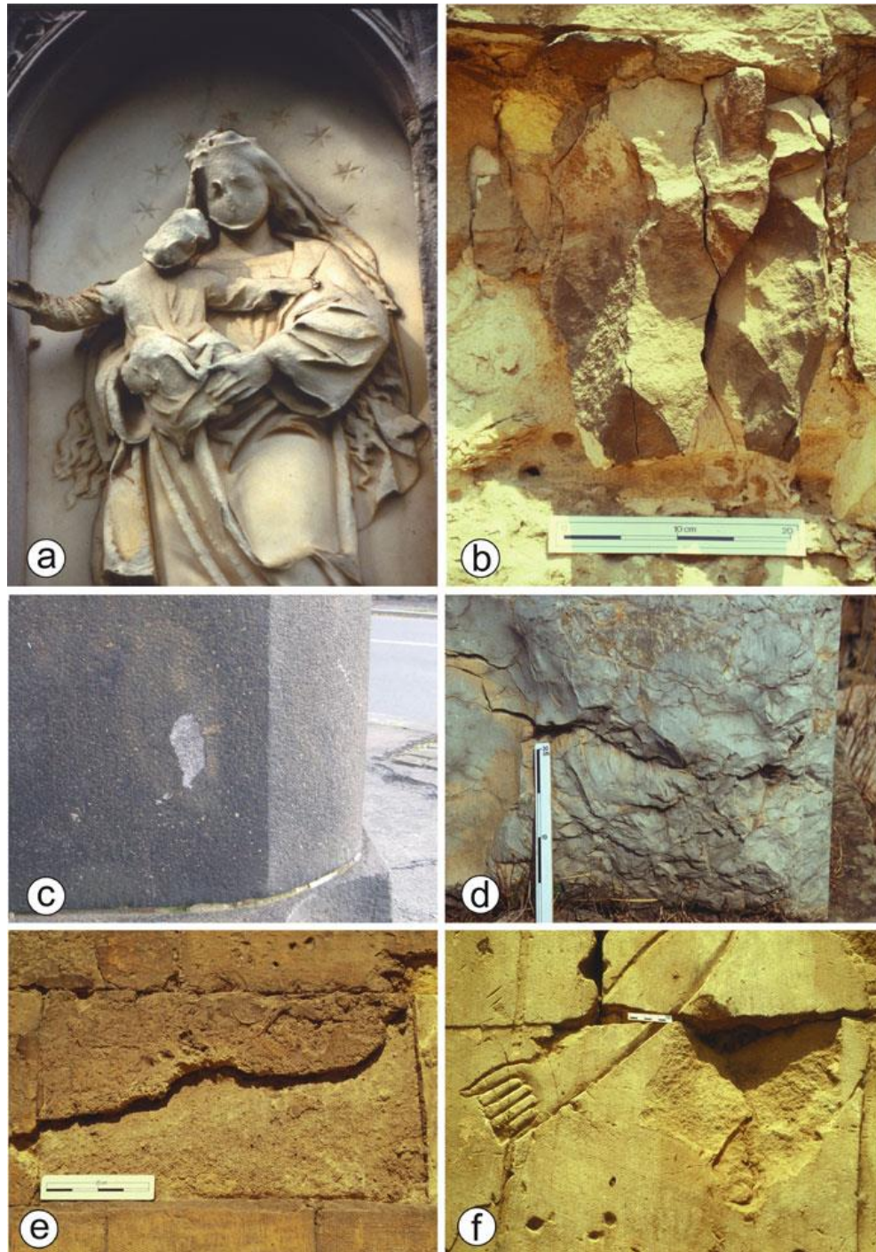
Figure 4.4 Detachment 2: (a) disintegration – marble sugaring (Germany), (b) disintegration – crumbling on limestone (Egypt), (c) blistering on granite, (Germany) (d) fragmentation - splintering on limestone(Greece), (e) contour scaling on limestone (Egypt), and (f) bursting on sandstone (Egypt) (Siegesmund & Snethlage, 2011)
