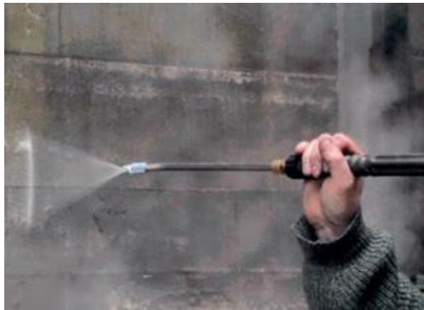
Figure 4.13 A large steam cleaner being used to clean ashlar with a 45° fan nozzle
