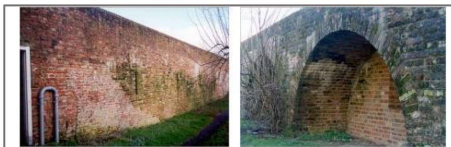
Figure 2.17 Examples of the growth of algae on masonry monuments
