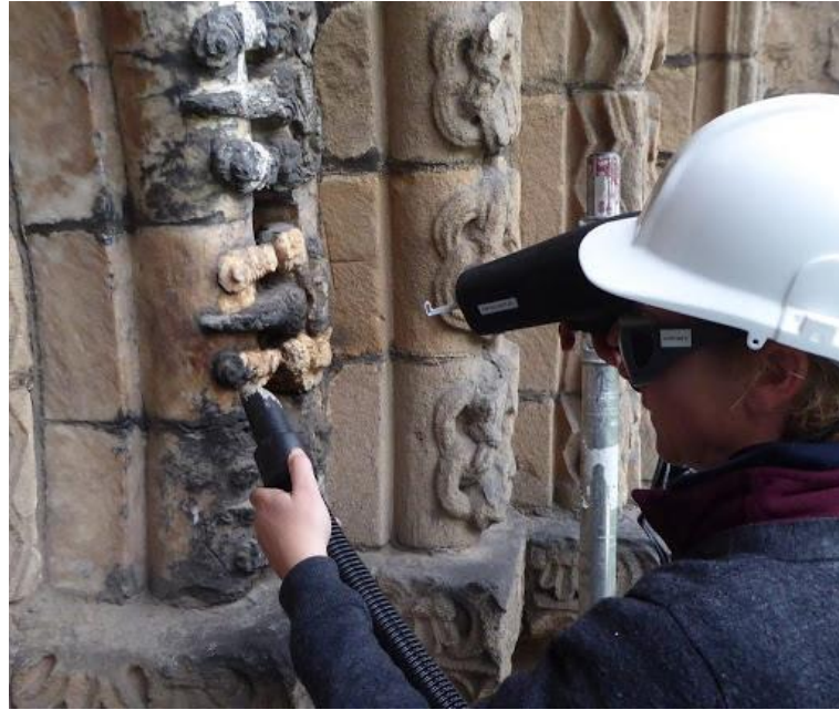
Figure 4.17 Application of mechanical cleaning
