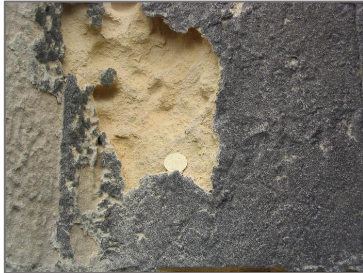
Figure 2.10 Granular disintegration on St Etienne church, Fécamp, Seine-Maritime, France (limestone). This church is located 300m of the sea (Angeli, 2007).
