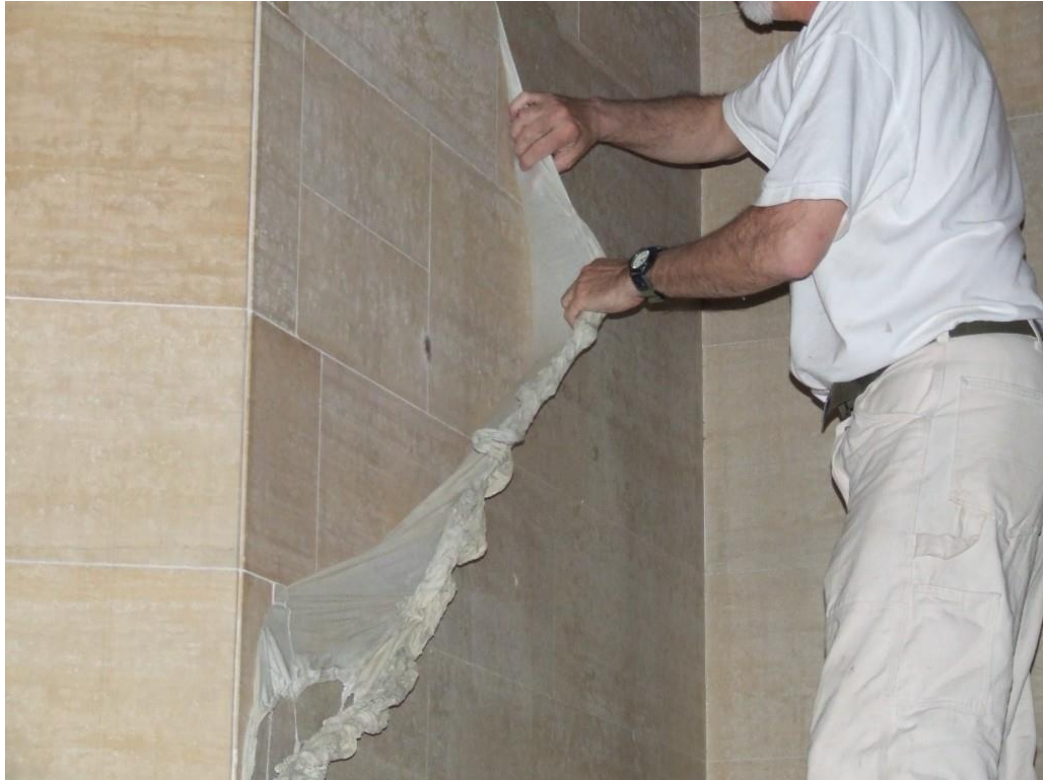
Figure 4.15 Removal of poultice
