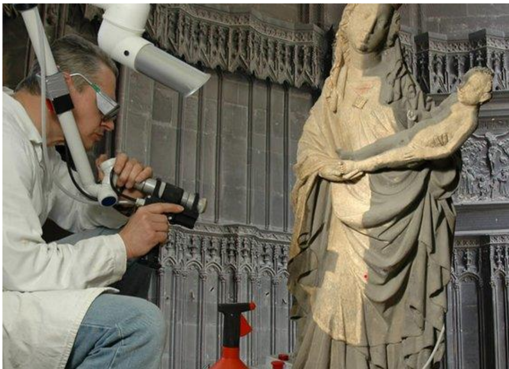
Figure 4.18 Stephan's Cathedral was laser cleaned with 30,000 hours of work in 7 years. Despite the long workforce, it has been calculated that it is less costly than cleaning applications that can be done with traditional methods due to reasons such as the large number of details in the building and its spread over a wide area.
